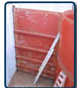
IN PROGRESS: Retrofitting with dewaterable partitions.
