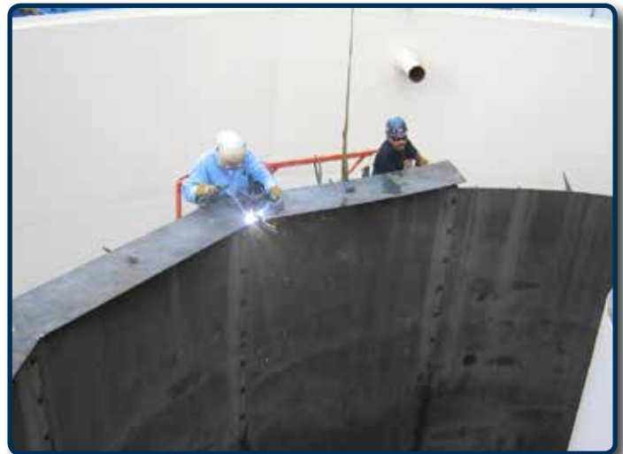
IN PROGRESS: Retrofitting bottom of the effluent trough.
