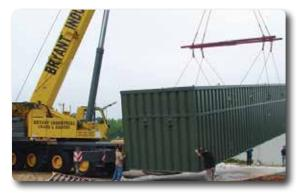
Offering minimal shipping and installation costs, **TITAN QUBE™** system arrives at the site wired with all components except power and pad. Simply place screen, connect main power and influent/ effluent pipes, raise junction boxes and you are ready to go.
